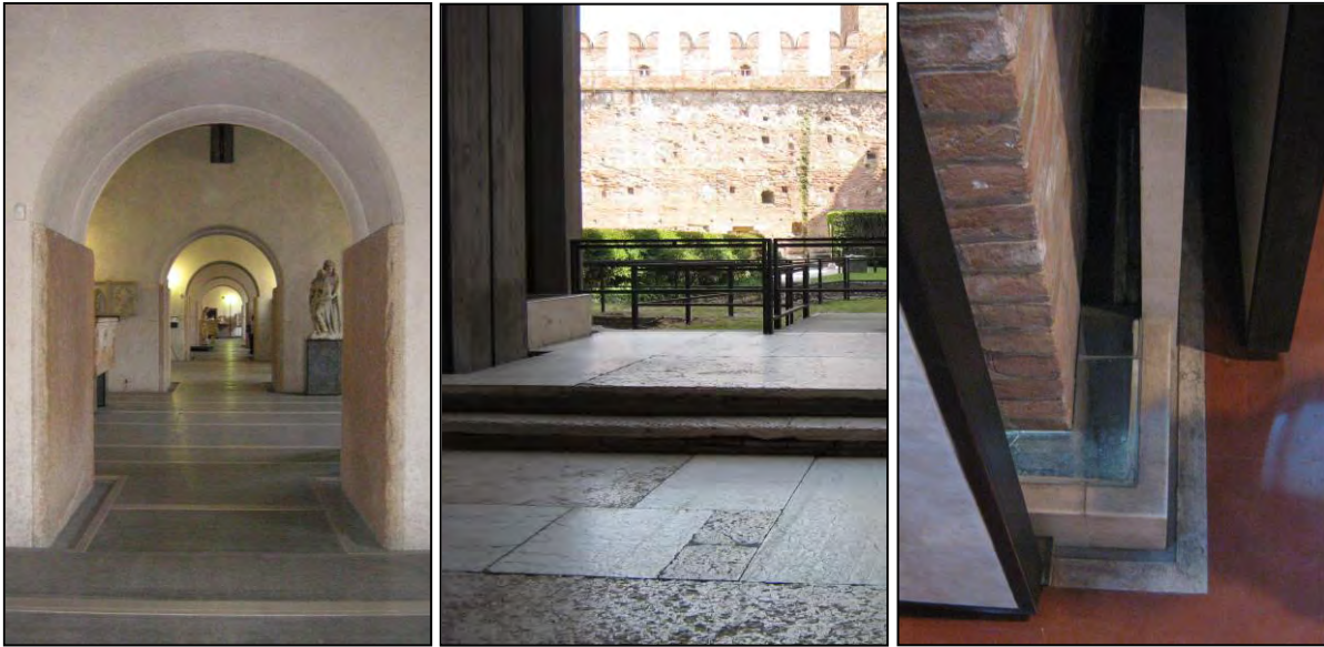
Figures 20 - 22: Floor slabs in the Castelvecchio: Verona, Italy
